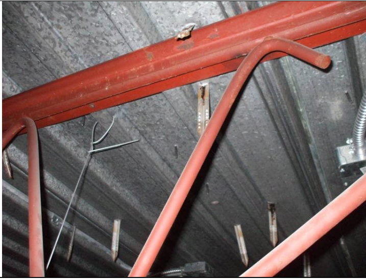
PHOTO 4 – EXAMPLE OF UPPER ROOFING MATERIAL.
